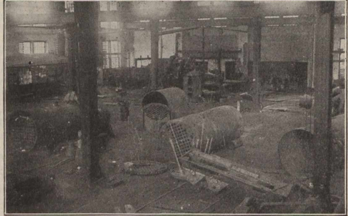
Fig. 6.—Boiler and Tank Shop Floor.
