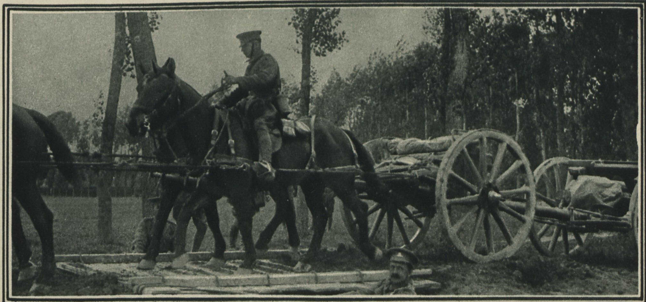
ARTILLERY CROSSING THE BRIDGE
