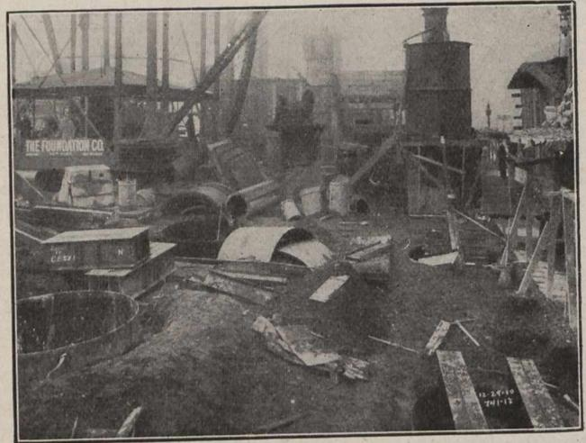
Fig. 4. Showing work on December 29, 1910, with grillage on Caisson in foreground.
