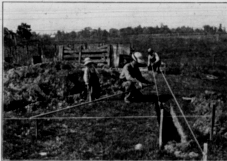
Securing up the foundation for a farm building, using six feet on one side, eight on the other and ten feet across.
