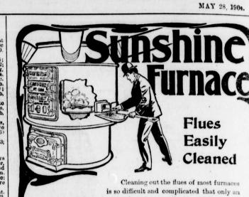
expert can do it, and experts' services usually come high. The flues in the Sunshine Furnace can be cleaned from two different clean-out doors and from the feed-door, so that there is no part of the flues which is not easily reached.
