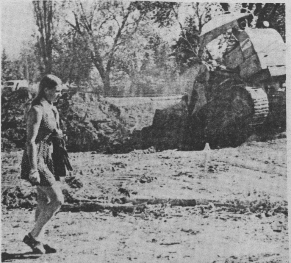
Construction began in October on the new Housing Union Building (HUB).
