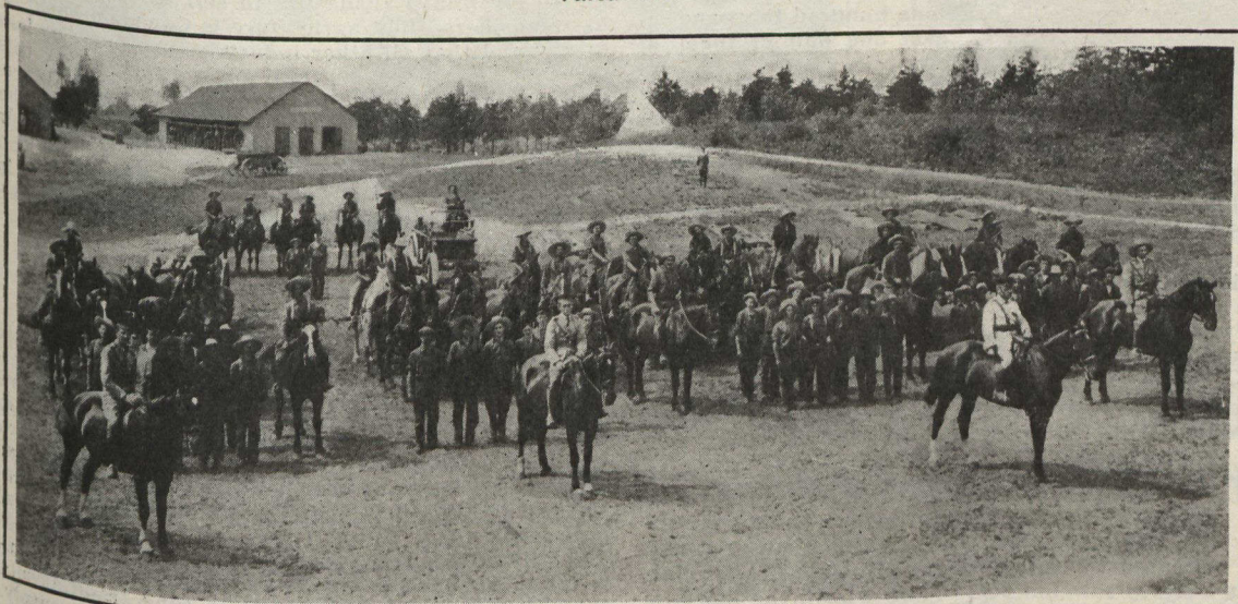
In 24 hours Cobourg heavy battery of artillery was mobilized; 24 hours later in camp at Beaumont, P.Q.; 24 hours again and it struck camp, and was ready to move in 90 minutes for the Pacific Coast via the C. P. R.
