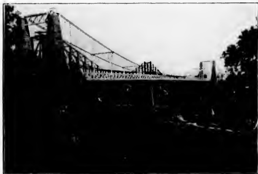
The Bridges, St. John.
