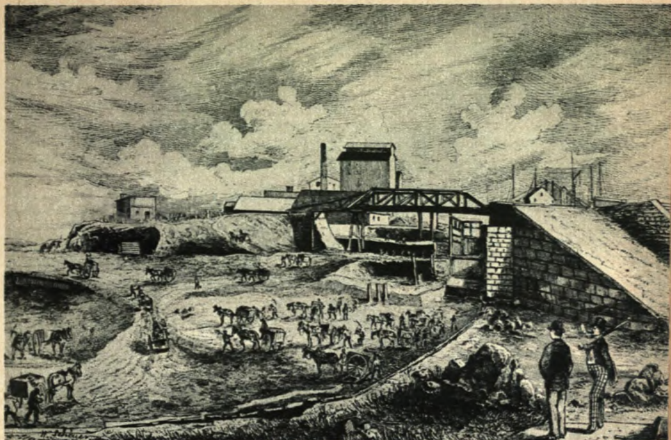
Early excavation operations on the old Lachine Canal connecting the Port of Montreal and Lake St. Louis
