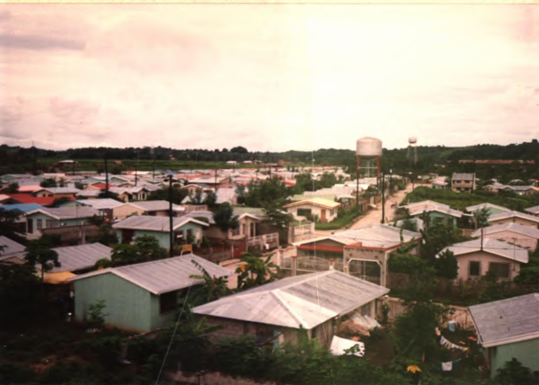
No. 60. "Pacita Complex". A 7,000 home subdivision financed by GSIS and constructed by a private builder. All houses are of hollow cement block.
