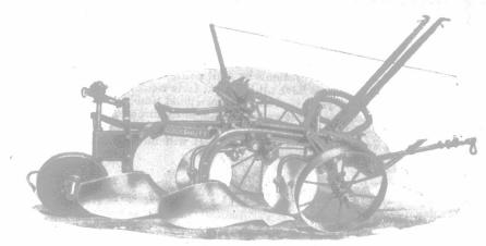
Cockshutt 2-Furrow Ligh: Tractor Plow---can be quickly turned into a 3-Furrow Plow by the addition of a few parts
