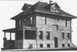
Note the Artistic Effect of "Ideal" Blocks in Residence Construction.
