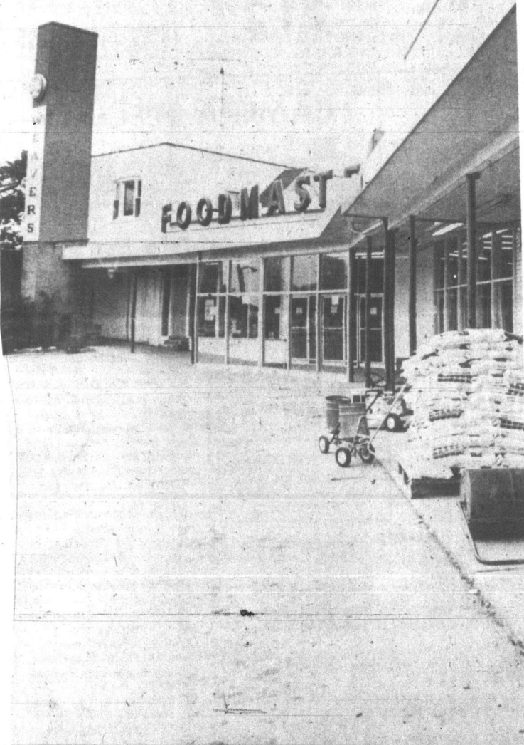
The new Weavers combines food market with hardware and garden centre. Future plans call for new market and complete home centre.
