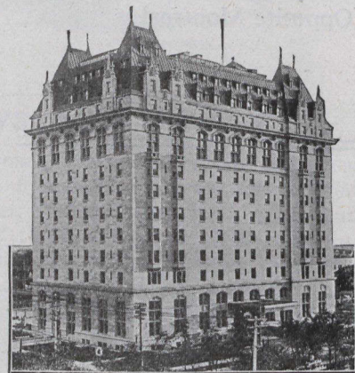
Fort Garry Hotel, Winnipeg. Arch: Ross & MacDonald, Montreal. El. Cont: L. E. Nielson Co., Inc. Pittsburgh.
