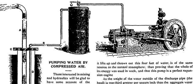
Pohlé system of raising water from non-flowing wells, mines, etc., which has been introduced into Canada by the Ingersoll-Sergeant Drill Company of Montreal
