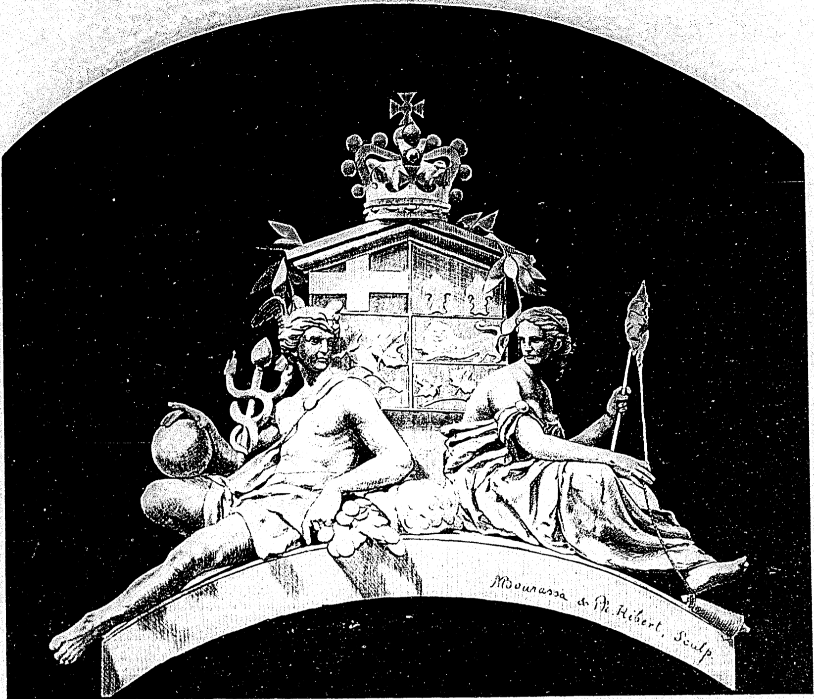
MONTREAL :—GROUP, REPRESENTING COMMERCE AND INDUSTRY, ERECTED ABOVE THE PEDIMENT OF THE NEW POST OFFICE.
