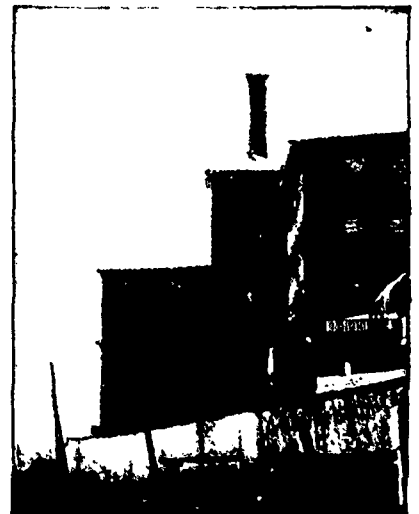
The same Chimney AFTER the American stoker was installed.
