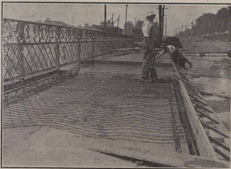
Fig. 11.—Method of Reinforcing Sidewalk Slab.
