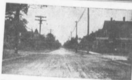
Two-course concrete street, Amherst, N.S., laid in 1914.
