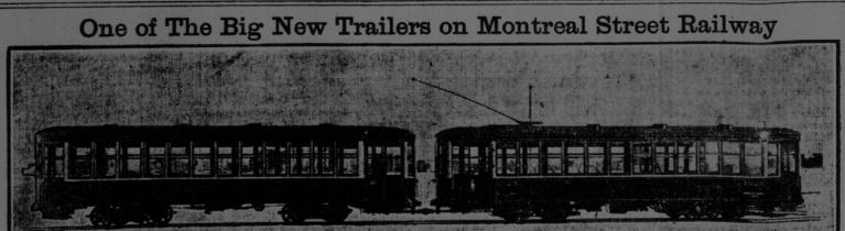
For a long time Montreal has been experimenting with a new style of street car trailer, and the public as well as the company think it a great success. The picture shows the trailer the same size as the motor. The conductor lowers the step by means of a lever, and in this way the car is picked up as it were, when in motion, thus preventing accidents, from boarding cars in motion.
