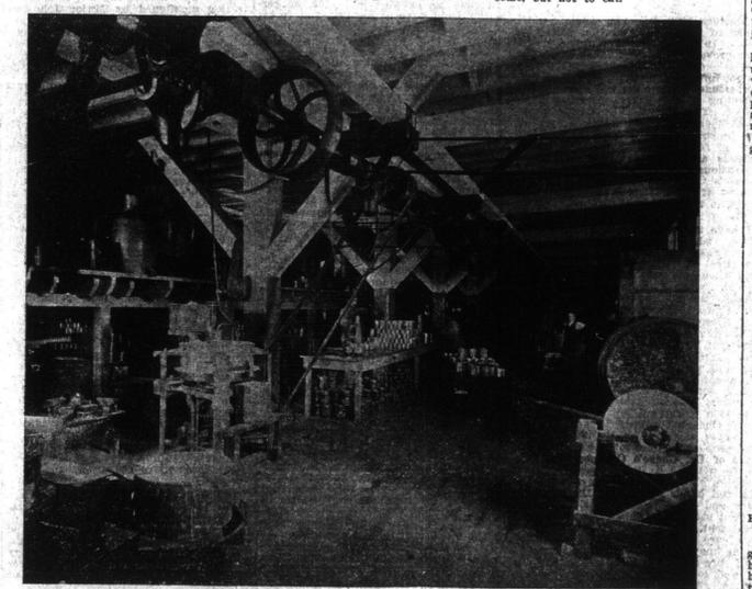
LIQUID PAINTS AND COLOR GRINDING DEPARTMENTS — GRINDING MACHINERY IS AT FAR END OF FLOOR. AND IS FED BY CONDUITS FROM MIXING MILLS ON FLOOR ABOVE.
