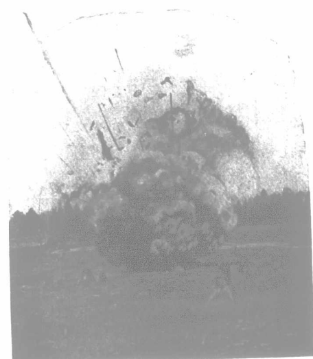
This cut shows how stumps are removed by using our new explosive.
