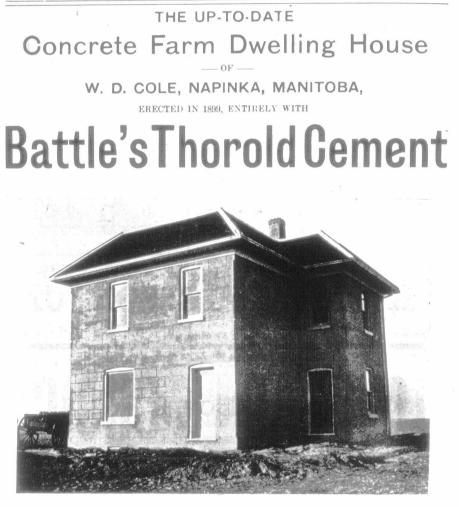
Foundation 30 x 32 feet. Basement walls 7 feet high and 1 foot thick. First storey 9 feet high, walls 10 inches thick. Second storey 8
