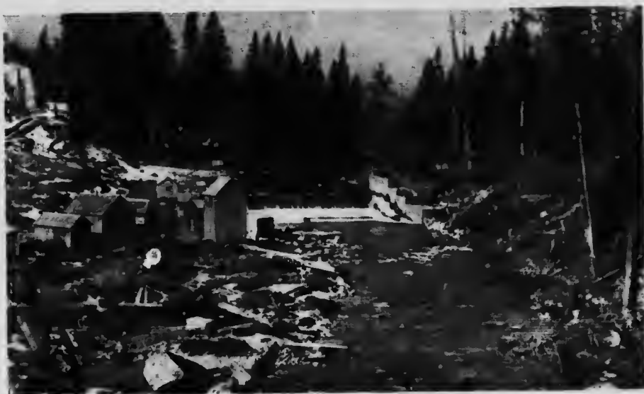
Coquitlam-Buntzen Development. Old Crib Dam, Coquitlam Lake.
