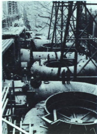
Power house under construction at the Warsak project in Pakistan.
