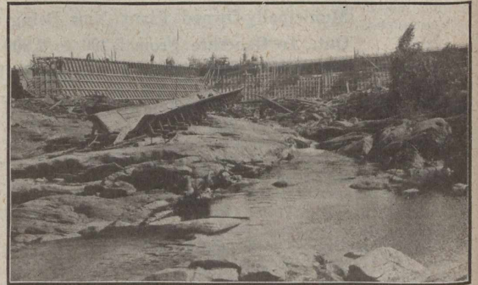
FIG. 5—NEW POWER DAM, LOOKING UP-STREAM
