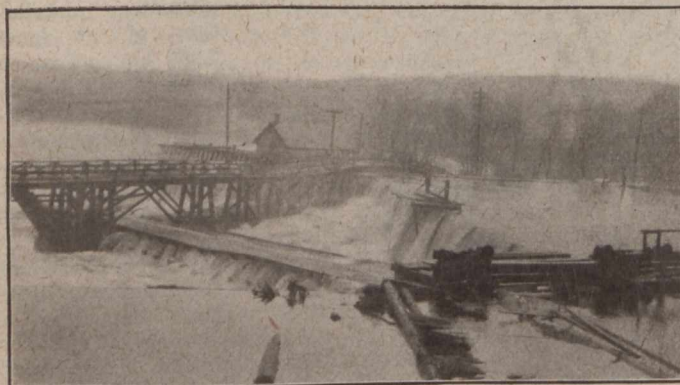
FIG. 4—OLD DAM AND HIGHWAY BRIDGE, LOOKING DOWN-STREAM
