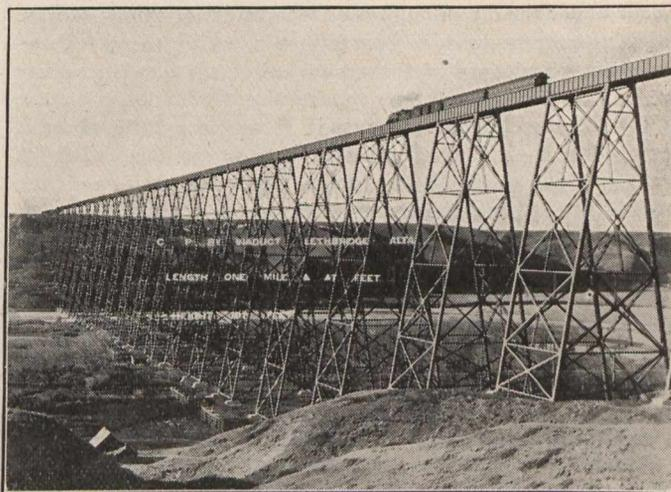
11 inches, and a height above the water level of 118 feet. It consists of four deck spans each 210 feet in length with a 40-foot plate deck girder between each, and a 60-foot plate deck girder at each abutment.
