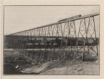
11 inches, and a height above the water level of 118 feet. It consists of four deck spans each 210 feet in length with a 40-foot plate deck girder between each, and a 60-feet plate deck girder at each abutment.
