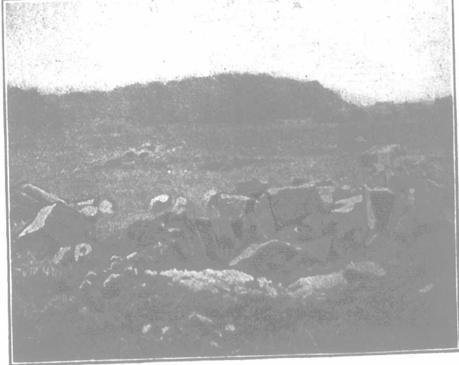
What happened to the boulder by using Stumping Powder.
