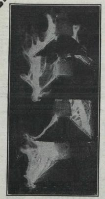
HOWING four "Victor" Suspension Insulator Units under severe rain test at 205, 000 volts; also a 65-ft. steel tower equipped for 100,000-volt operation. This is part of an experimental tower line at Victor, 800-ft. span, running up to 350,000 volts.
