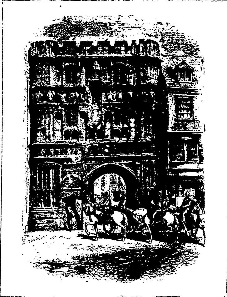
PRECINCT GATE, CANTERBURY.
