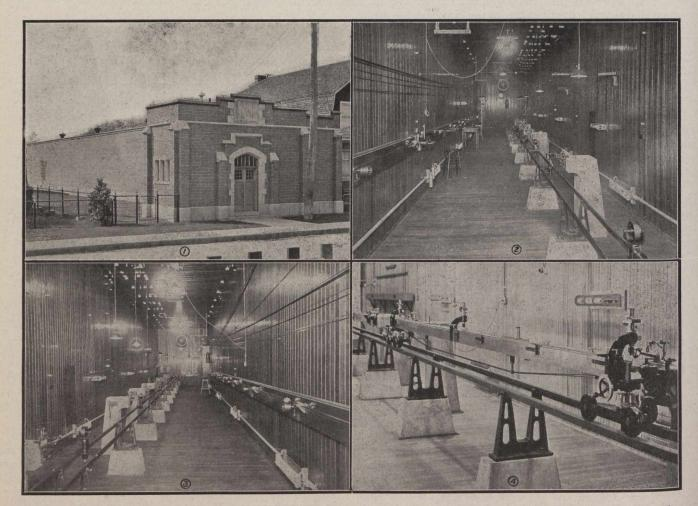
Fig. 1.—Exterior, Comparator Building; Figs. 2 (and 3).—Interior of Tape-testing Room, Looking North (and South); Fig. 4.—Meter Invar Bar in Position for Reading.
