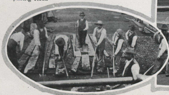
Laying Concrete Pavement
