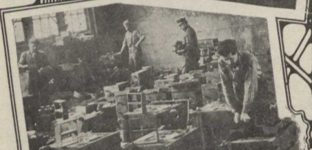
Cylinder Casting Room
