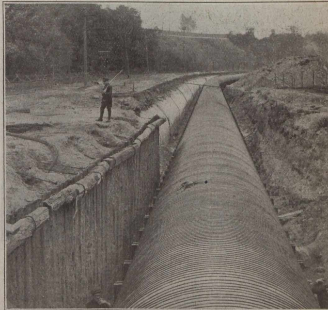
NO. 3 CONDUIT COMPLETED, SHOWING METHOD OF BRACING LACKAWANNA STEEL SHEET PILING BETWEEN CONDUITS NOS. 2 AND 3
