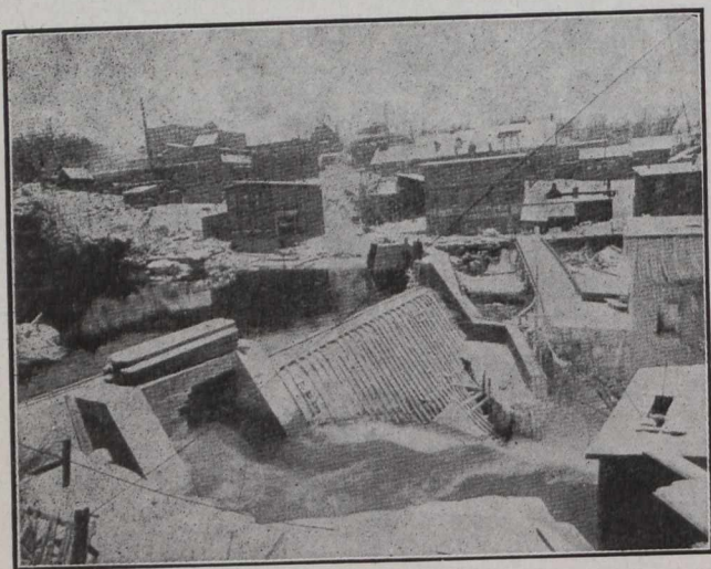
View showing ice formation on walls of factory, (while flow of river was being passed over the old head-race wall).
