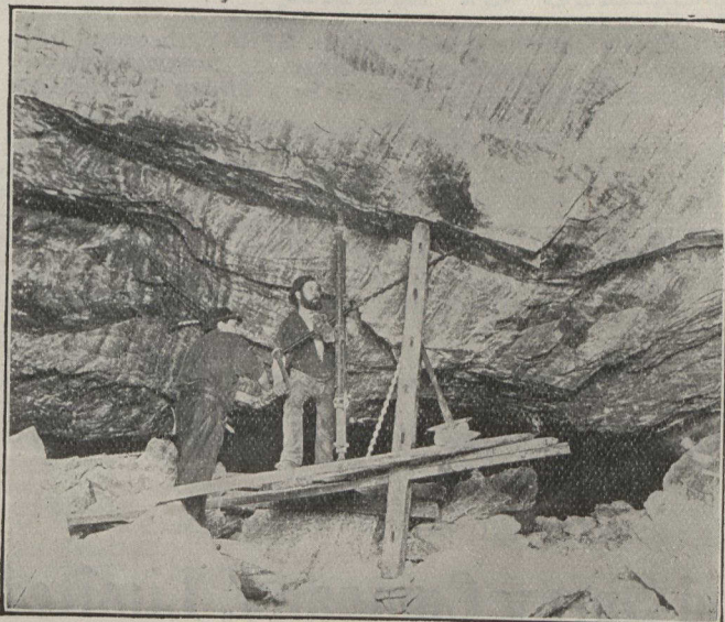
Drilling for Blasting
