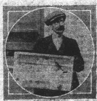
This is the method adopted by England to test the atmospheric conditions of coal mines. The picture shows a miner with a caged canary, which is lowered into the shafts to test the state of the poisonous air.
