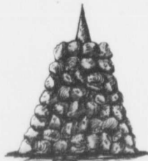
Inner Leading Beacon, North East Hill, Winter Harbour
