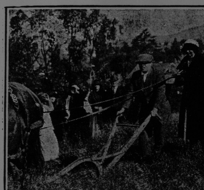
Aubrey Warden was a lineman employed by the Whittier (Calif.) Telephone company. He invested money in California's fabulously rich Santa Fe oil field. Now he is president of the telephone company, and this picture shows him breaking ground for the $100,000 dormitory he is erecting for Whittier College.
