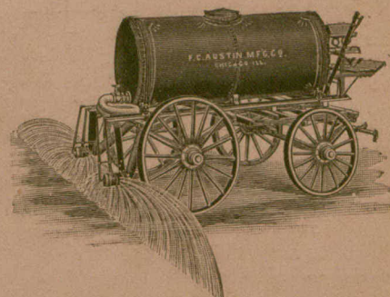
AUSTIN STEEL STREET SPRINKLER
