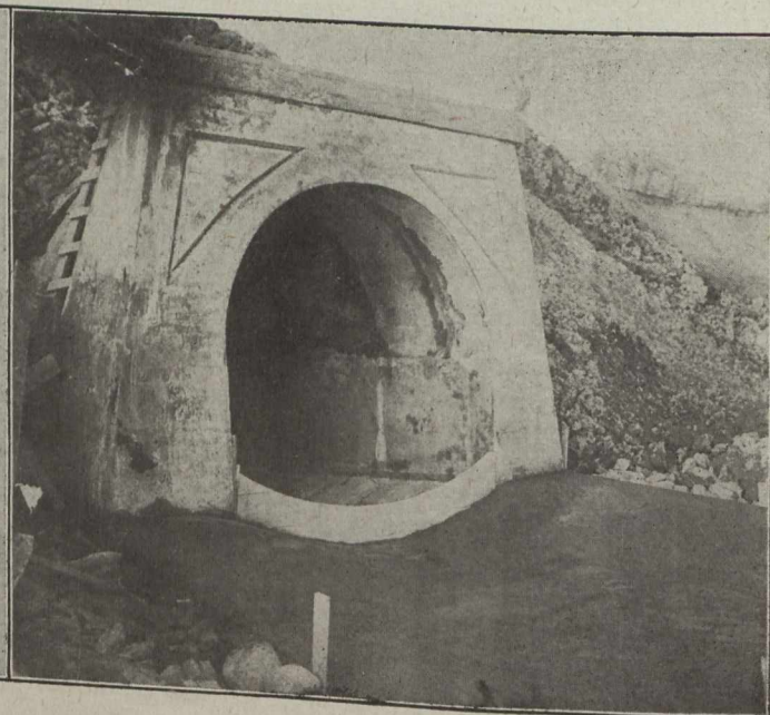
Fig. 7.—Outlet of Main Garrison Creek Storm Overflow Sewer at the Foot of Strachan Avenue.
