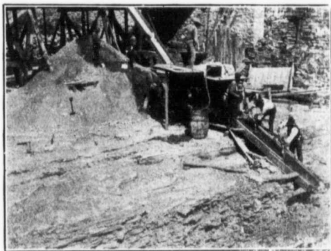
Fig. 1—Concrete Mixer at Work. 75 to 100 Tons per Day.
