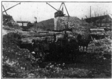
Fig. 2—Excavating for Heavy West Retaining Wall.
