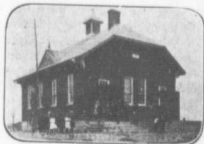
One Example of Progress
