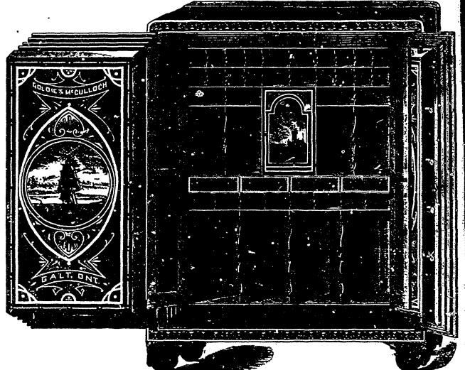
We have for more than a year past, prevented our Safe and Vault Door Locks from being drilled, by protecting them with a plate of DRILL PROOF STEEL. Although our Fire-Proof Safes are always filled with WET FILLING, we have succeeded, at considerable expanse, in perfecting their construction so as to effectually prevent their becoming Jamy, mouldy or musty inside, and our largely increasing sales are good evidence of the fact that the public appreciate these qualities.
