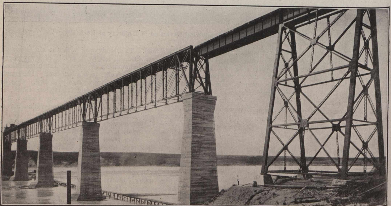
View of the River Section of the Outlook Bridge. At the Extreme Left is One of the Nine Land Towers.
