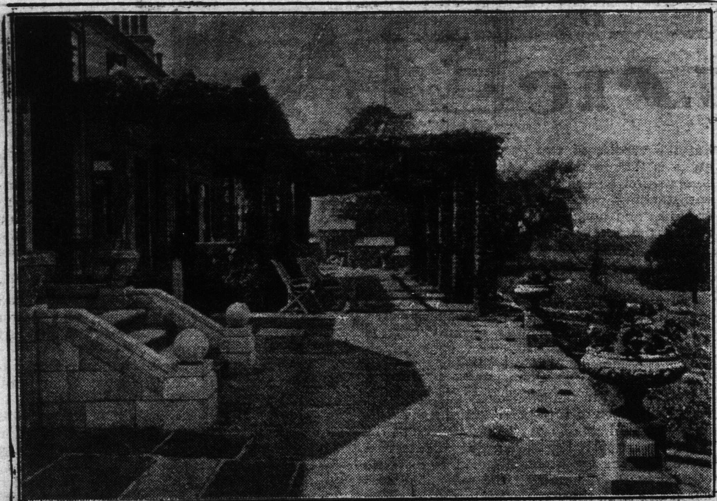
THE STONE TERRACE AND PERGOLA
