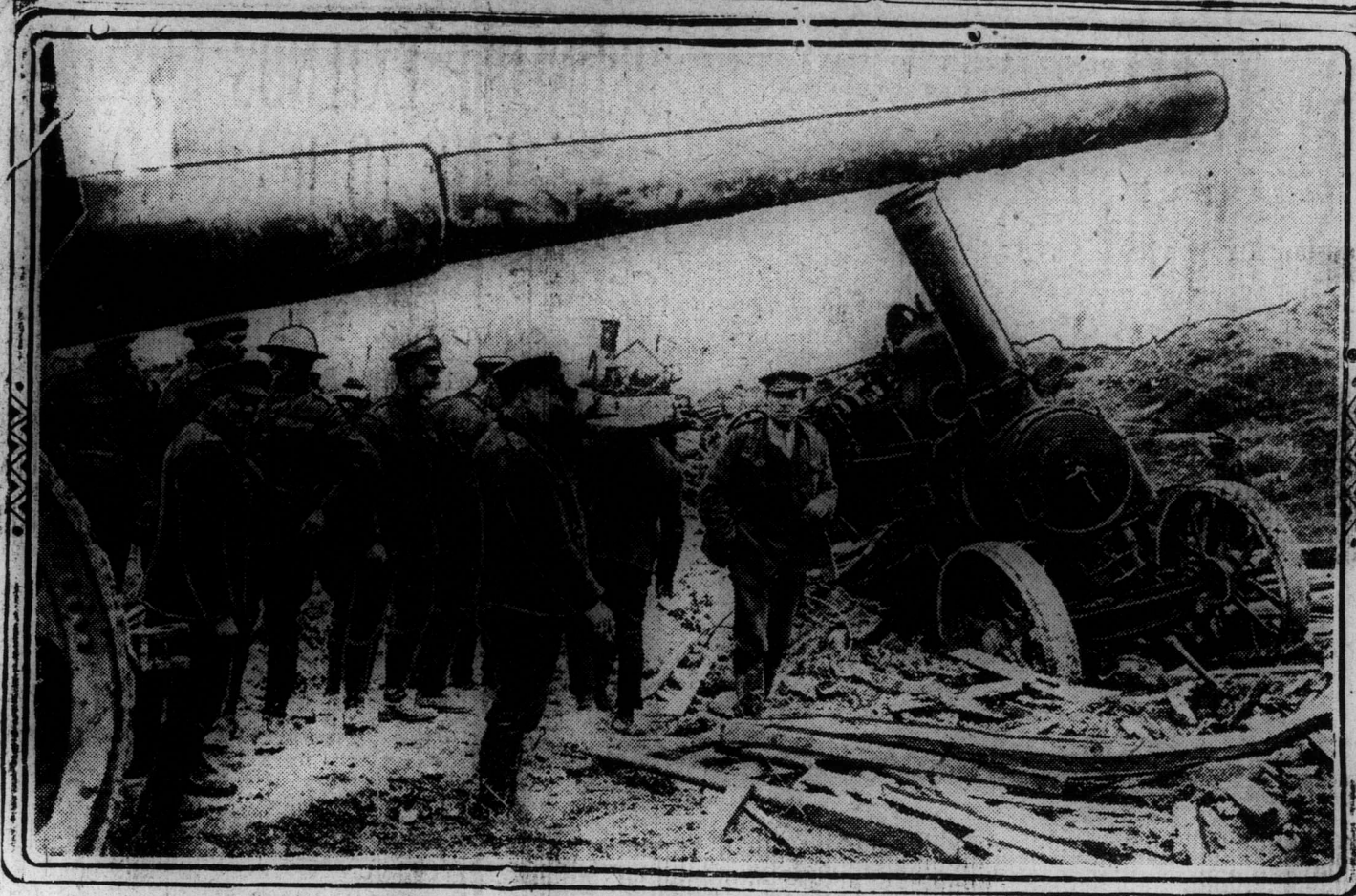
ONE OF THE BRITISH BIG GUNS THAT HAS SPOKEN A WORD OR TWO ON THE WESTERN FRONT British official photograph taken on the Western front. This monster British gun is being delayed in the advance because the tractor that hauls it forward has fallen into a rut and is disabled. Guns of this type have played a prominent part in the latest British advance. Their cooing words convinced the Germans that it is better to run than get hit.
