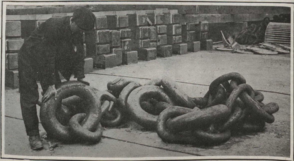
A few of the links in the great chain that will be used to tow the drydock.
