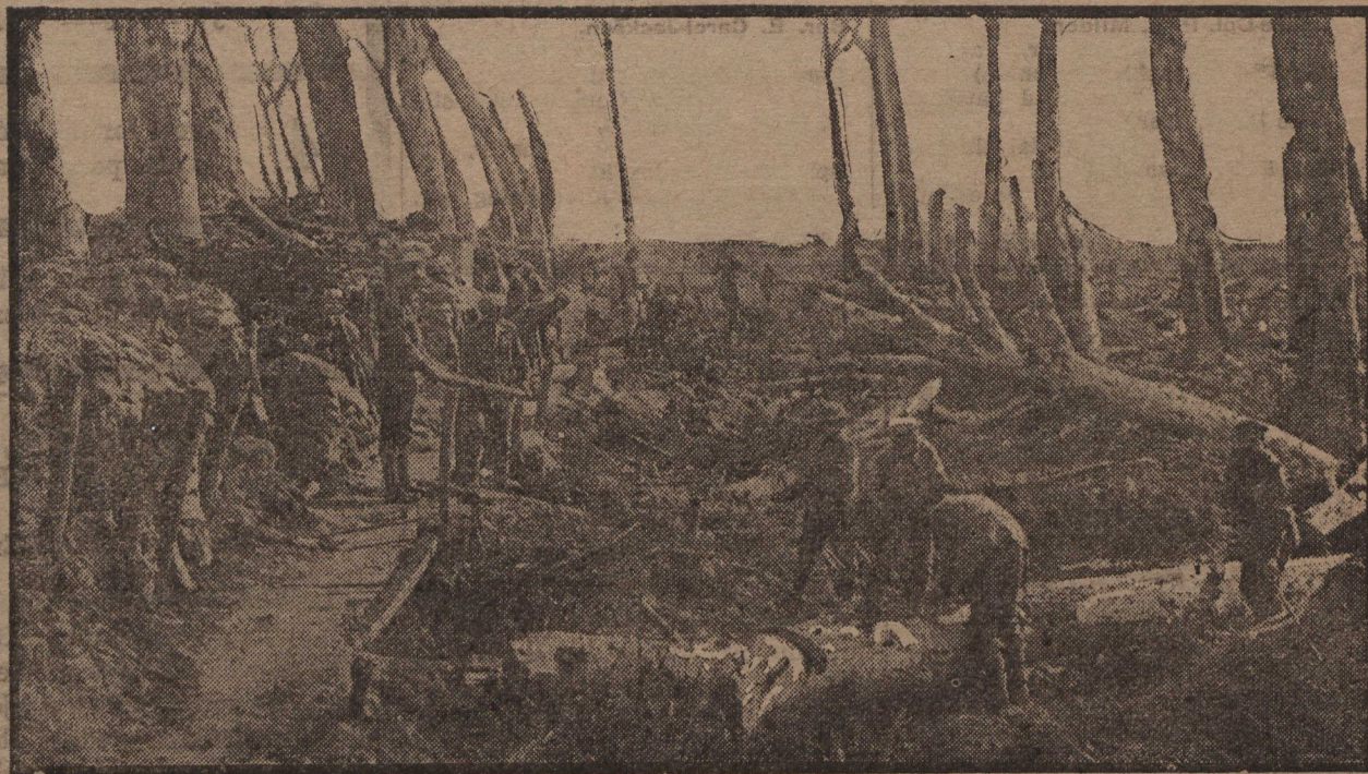
On the British Front in France.—Everything at the front is put to some use. These trees are being used for road-making and strengthening dug-outs.
